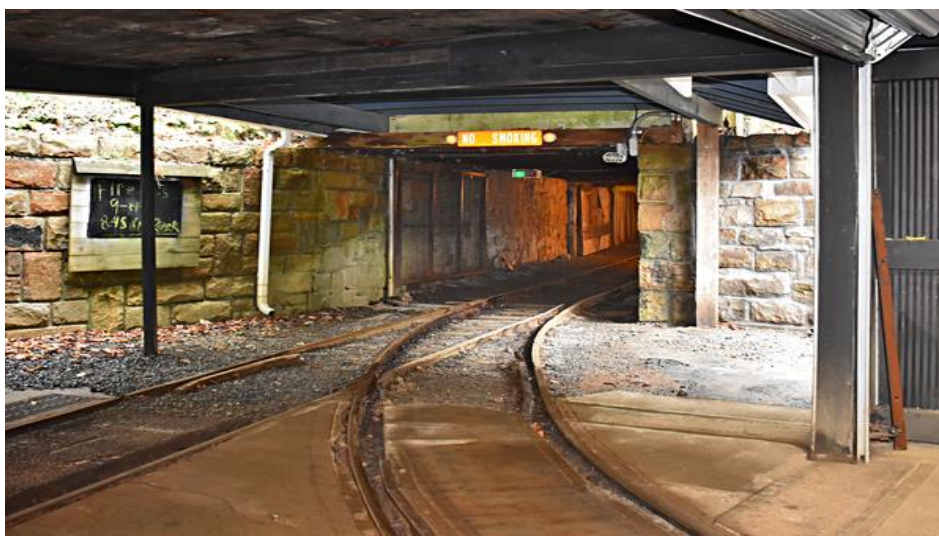
Figura 14. Big Bend Tunnel East
