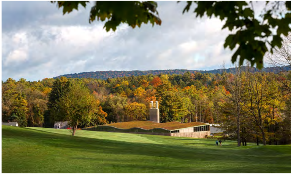
Figura 63 - Hotchkiss Biomass Powerplant
