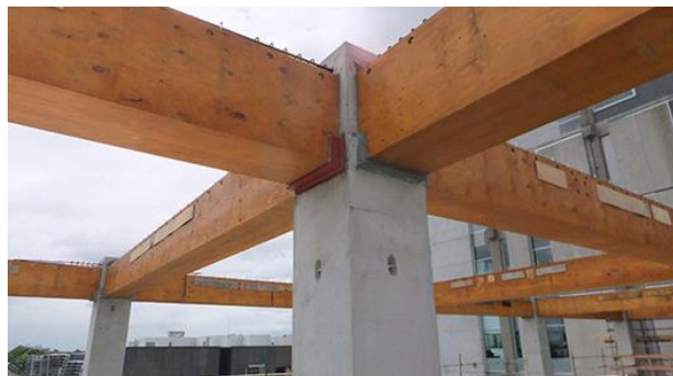
(b) hybrid joint: concrete-timber [30]
