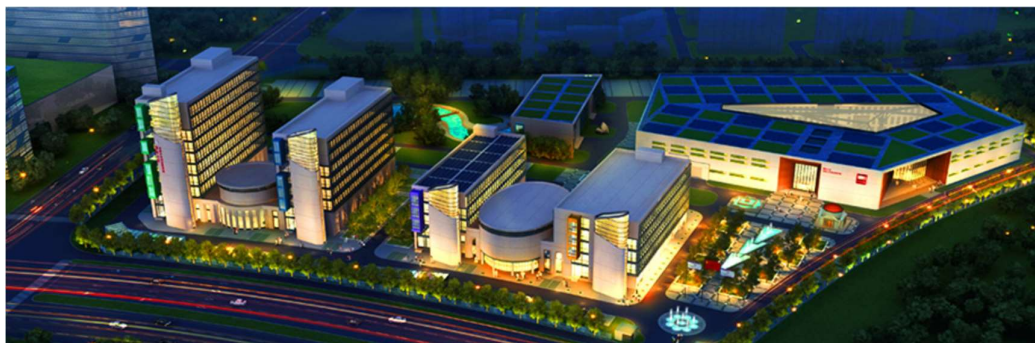
Figura 2.1– Vista geral de Hefei Instituto for Public Safety Research. Tsinghua University
