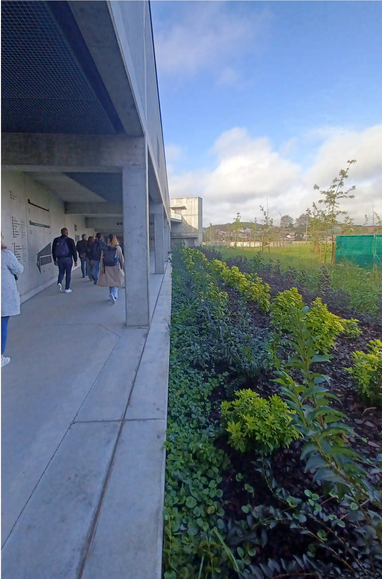
Figure 7: Photo of Campanhã Intermodal Terminal - Entrance coming from railway station.
