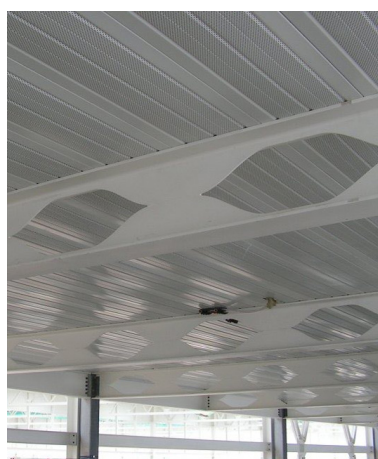
a) Angelina Beam – Arcelor-Mittal ; piso com solução Cofradal ( Arcelor-Mittal , 2013; Arcelor-Mittal , 2016).
