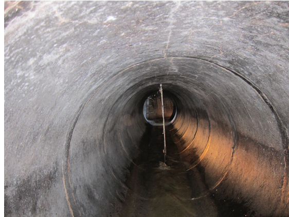
FIGURE 4.5: Interior of an underground conduit.
