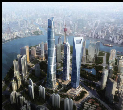
Fig.21 | Xangai WFC e Xangai Tower , Kohn Pederson Fox Associates e Marshall Strabala.
