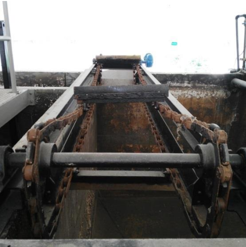
Figure iii. Metal blades of the first tank to remove the fats.
