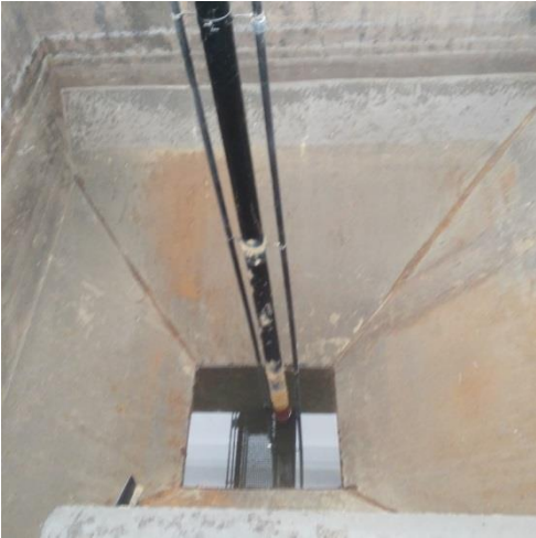
Figure ii. Bottom of the first tank where the muds are settled.
