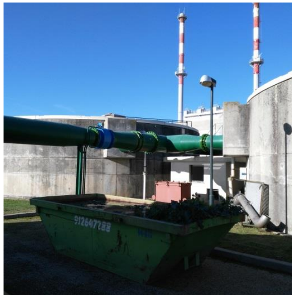
Figure iv. First decantation tank.
