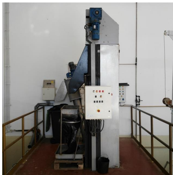
Figure i. Motor to remove big solids in the preliminary stage.
