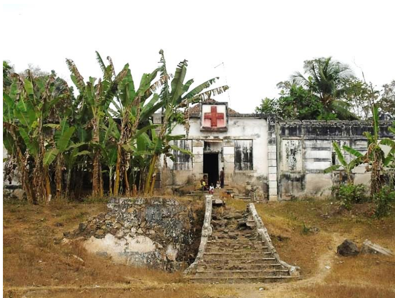
Figure 23 – Community of Plancas I. Abandoned hospital
