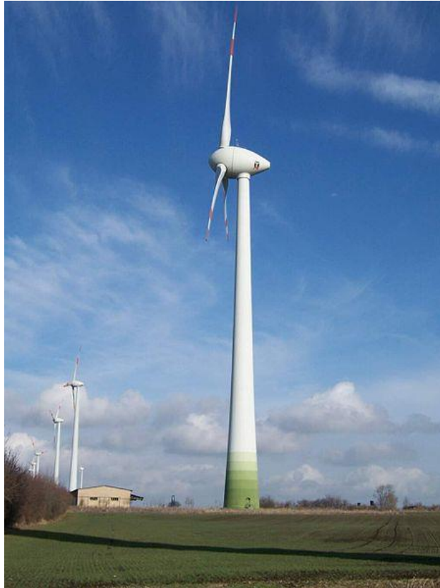
Figure 2.4 – Concrete tower prototype Enercon E-112
