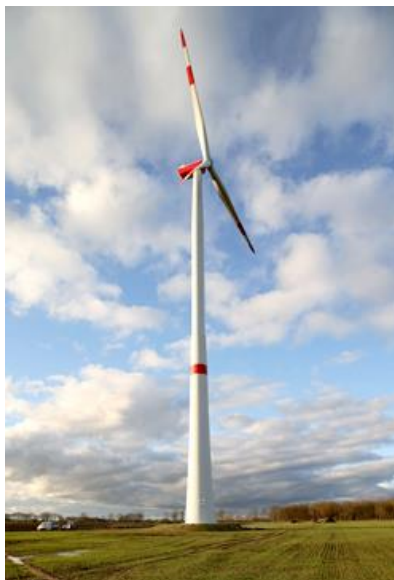
Figure 2.5 – Nordex turbine N90/2500 supported by 120 m hybrid concrete-steel tower
