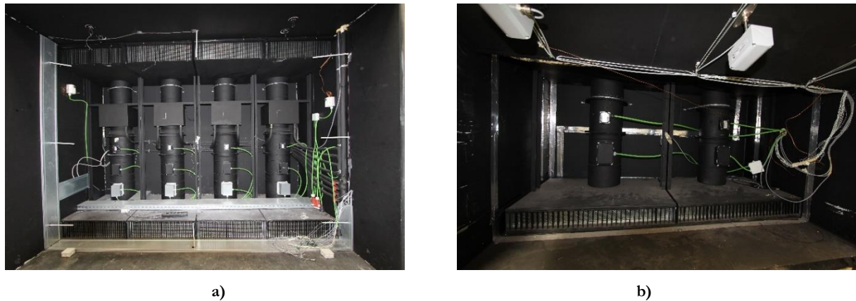
Figure 4.14 – Air circulation, heating and refrigeration system duct: a) guard/cold box; and b) GHB metering box.
