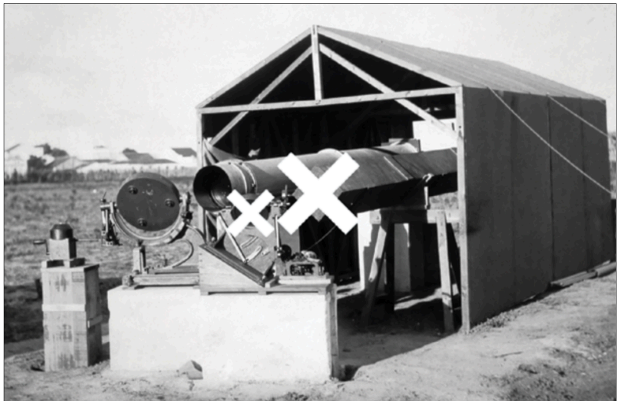
Figure 7: The installation at Príncipe was similar with that of Sobral but included just one telescope and a cœlostát, not the smaller telescope and cœlostát marked here with the crosses (Fotobanco Pao7TD; after Simões, 2019: 47).
