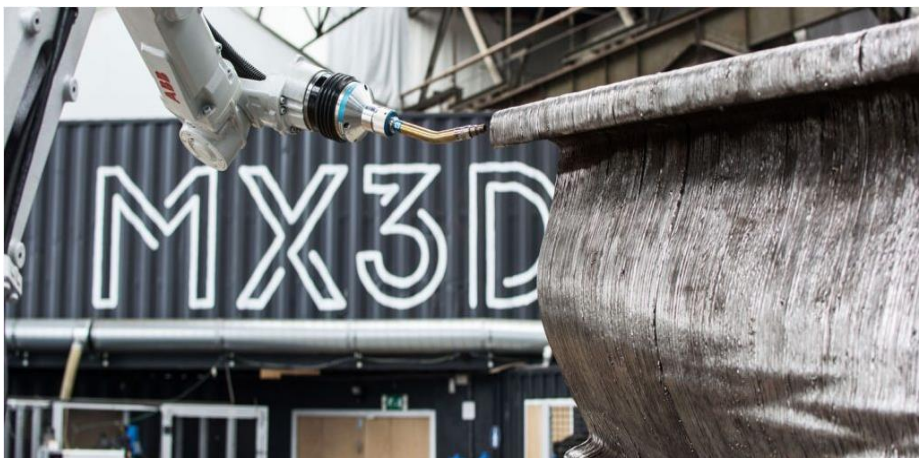
Figure 2.9 Horizontal Printing (MX3D Bridge | MX3D n.d.)
