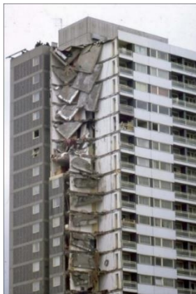
a. Ronan Apartment tower London
