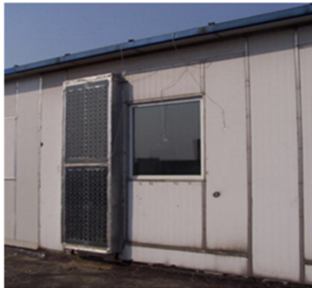
Figure 10 - Example of a photovoltaic Trombe wall (Saadatian et al. , 2012).
