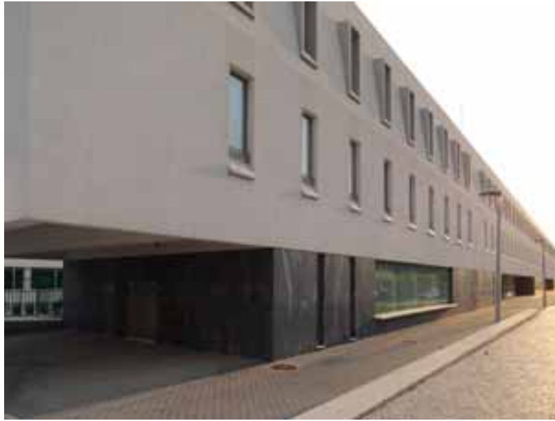
Fig. 145. Quinta das Flores School _ New building and its accesses from the street (Carolina Coelho)
