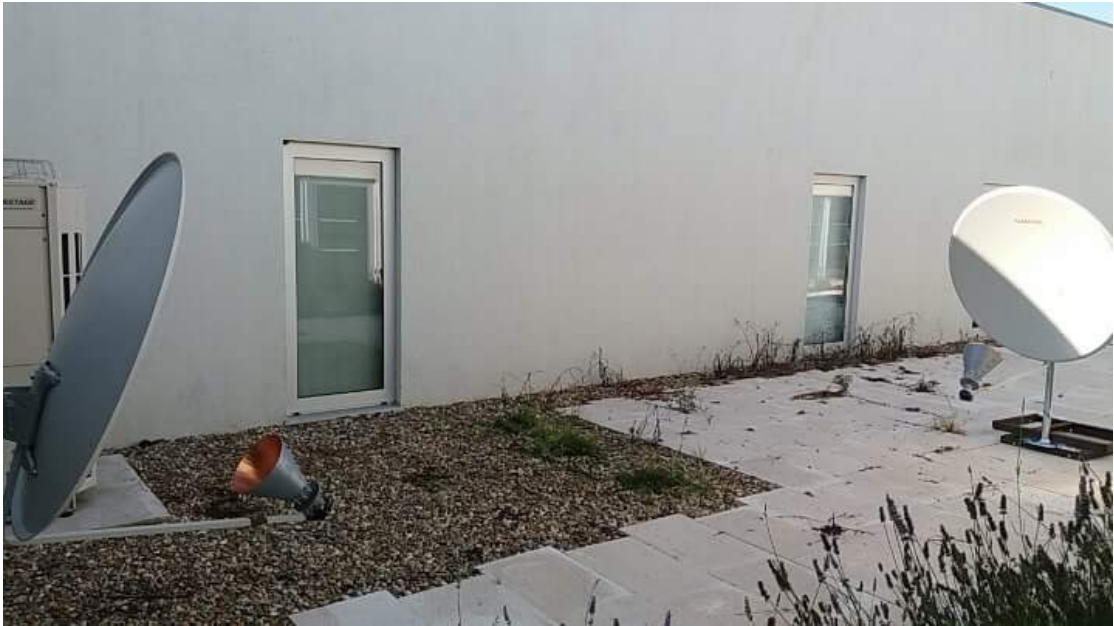
FIGURE 8.1: Emitter antenna and first parabolic reflector.
