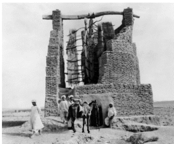
Figure 2.1 – Vertical-axis windmill for milling grain, Afghanistan (Deutsches Museum), (Hau, 2006)
