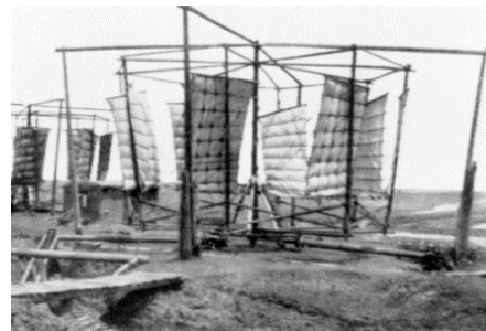
Figure 2.2 – Ancient Chinese windwheel for pumping water (Deutsches Museum), (Hau, 2006)
