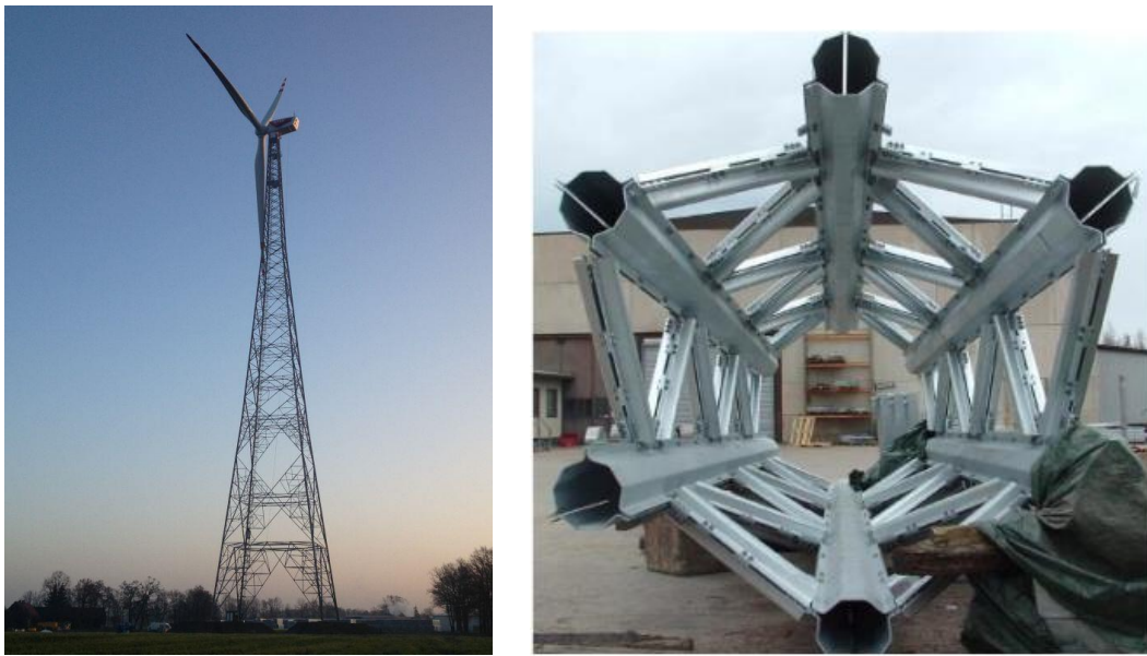
Figure 2.7: Lattice tower by Fuhrländer on left and by Ruukki on Right (epoznan.pt)
