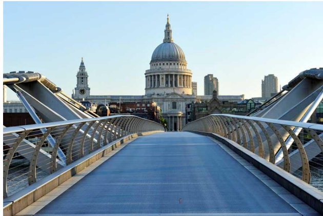
Figura 1 - Millennium Bridge, Londres (Fonte Nick Weall, Architecture Photography)
