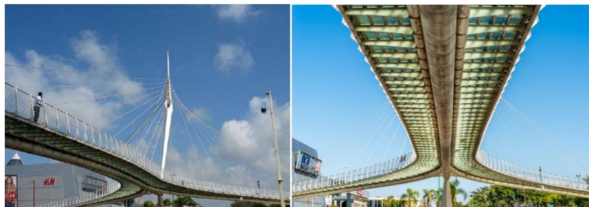
Figura 19 - Ponte Petah Tikva, Israel (Stankiewicz, et al., 2015)
