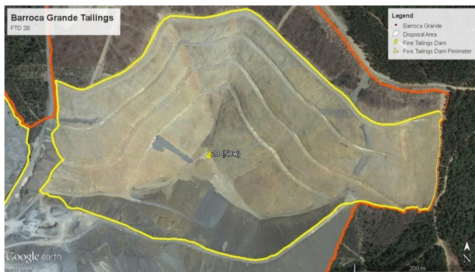
Figure 34 - Close-up view of the new fine tailings dam 2B as of May 2013 (Google Earth Pro version 7.1.5).
