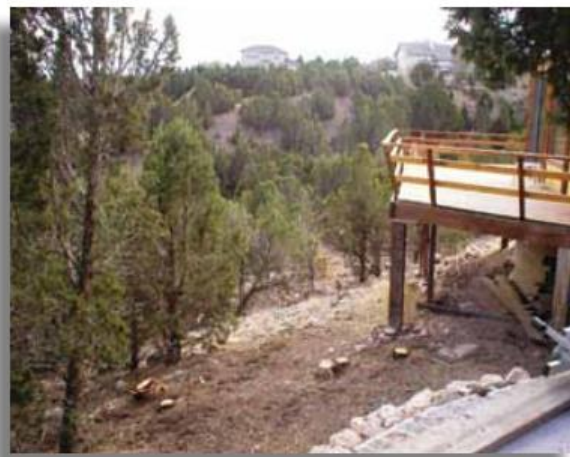
After mitigation work, deck is less likely to ignite
