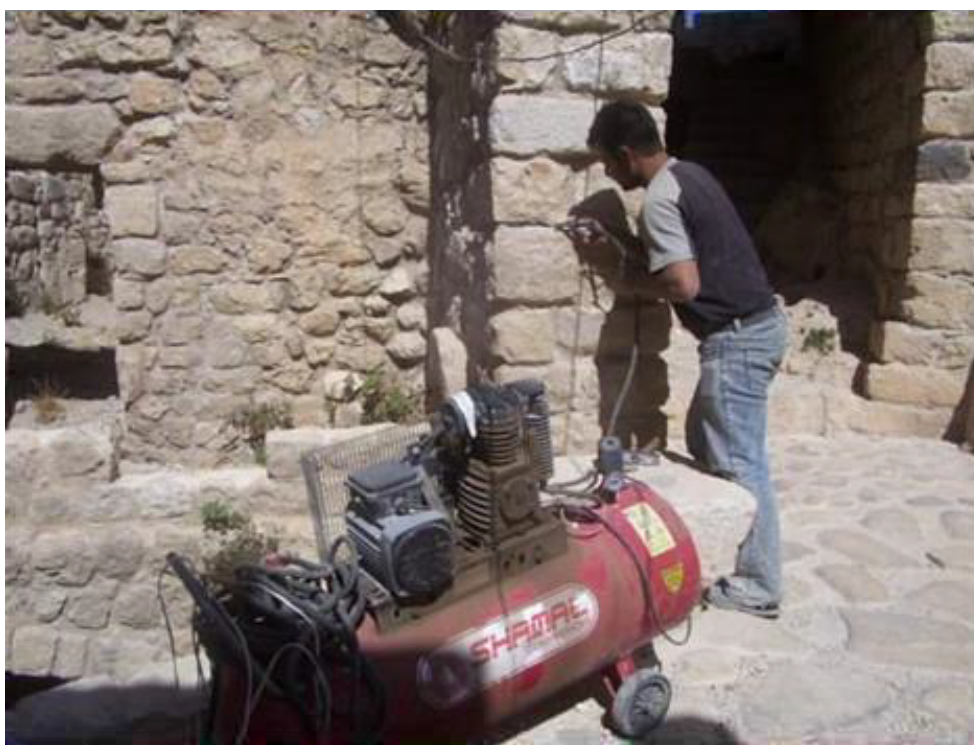
Figure: 10, using aerosol mist spray to clean the stone surfaces (Gonnella, 2008)
