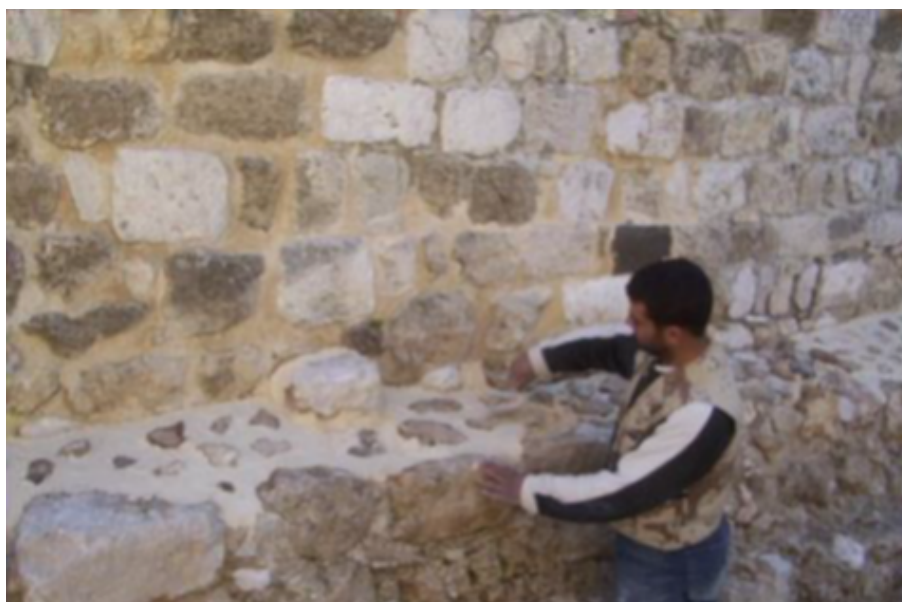
Figure: 15, the wall heads maintenance (AKTC, 2007)
