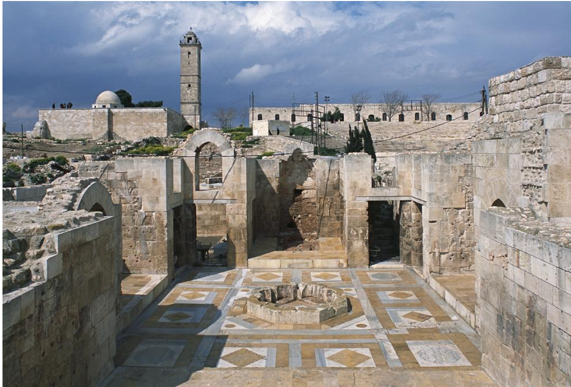
Figure: 6, the pavement of the Ayyubid Palace courtyard, after intervention 2003 (AKTC, 2007)
