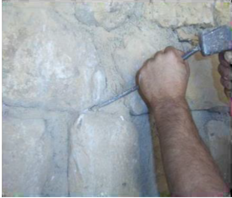
Figure: 3, removing the cement mortar (Culture, 2001)
