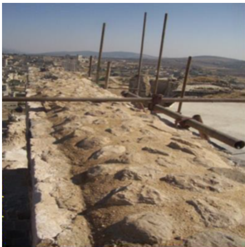
Figure: 14, the wall heads maintenance (AKTC, 2007)
