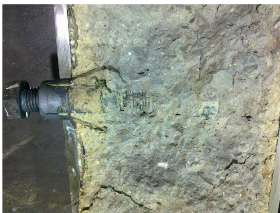
Figure 4.18. Specimen after fire exposure [97]
