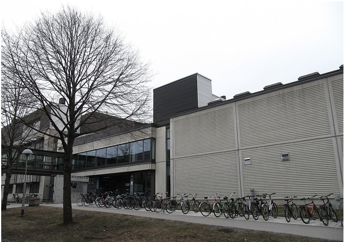
Figure 13 - Photo of the School of Architecture – Tampere University of Technology by Ana Moreira Bento
