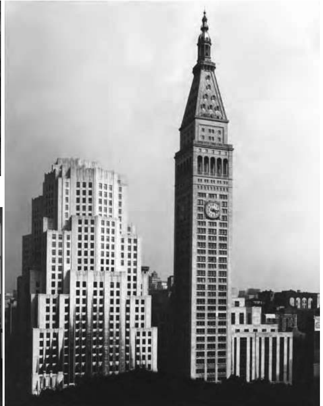
Figura 33 – Metropolitan Life Home Office Complex.
