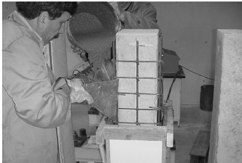
Fig. 6 Concrete casting of the jacket
