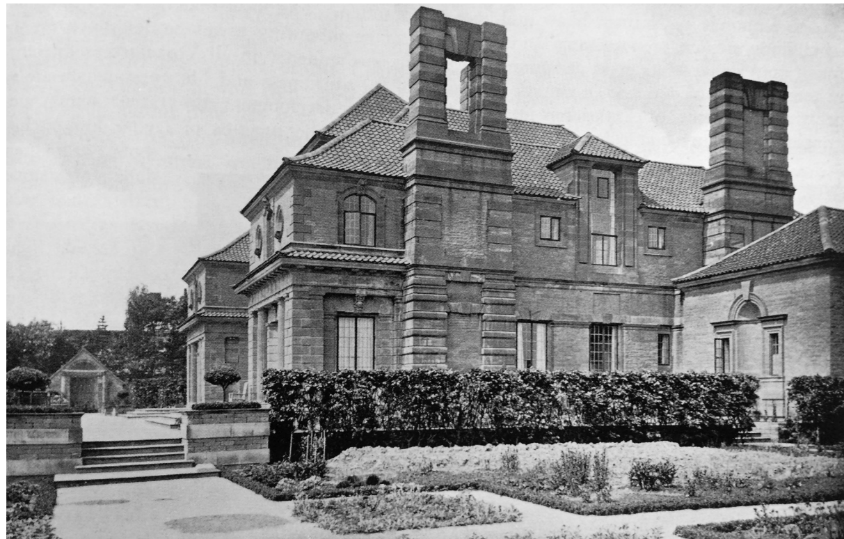
Heathcote: photograph of the east façade
