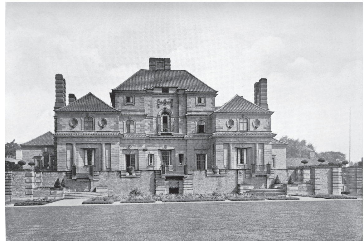
Heathcote: photograph of the south façade
