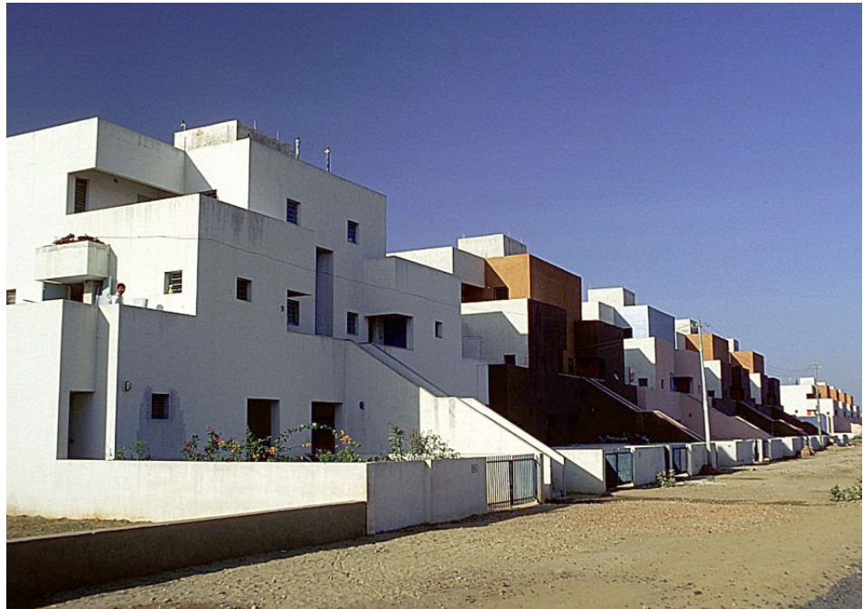
127. LIC Housing, Arq. Balkrishna Doshi, 1976, Ahmedabad, India.
