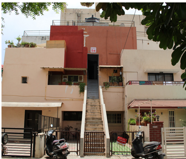
135. LIC Housing, Arq. Balkrishna Doshi, Ahmedabad, Abril de 2016.
