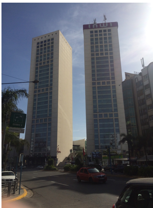
Figura 57 - Twin Center, Twin Towers, Ricardo Bofill
