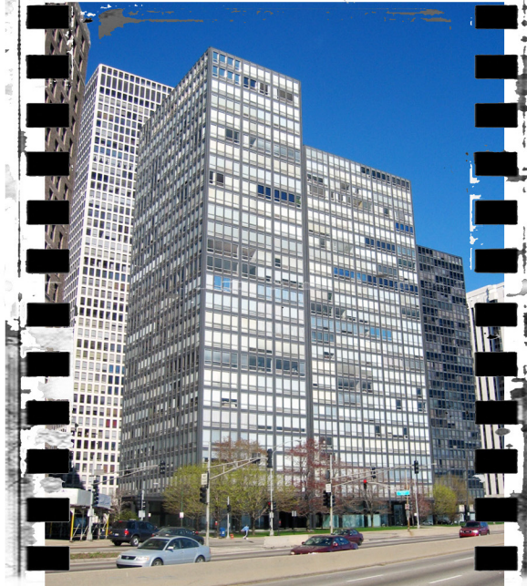
Seagram Building | Lake Shore Drive Apartments
