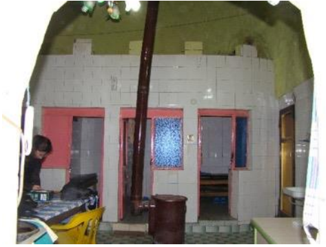
Figure 5 - rooms which are added later to Dünder Bey Bath
