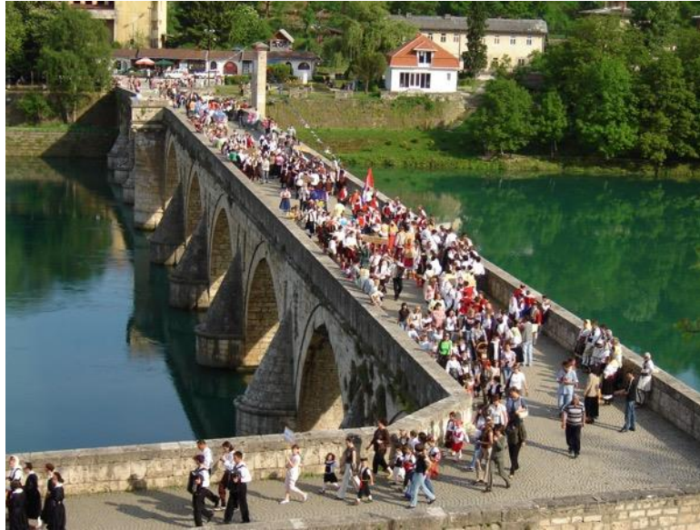
Figure 5 – Mehmed Paša Sokolović Bridge in Višegrad
