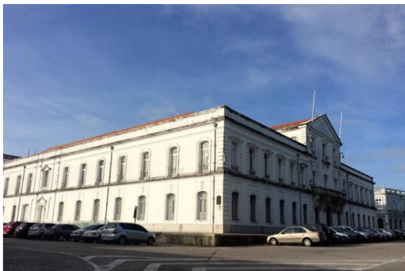
Figure 8 - Lauro Sodré Palace.
