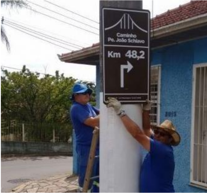
Figure 2 – Placing signs in the Padre João Schiavo route
