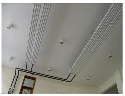
Figure 1.14. The radiant ceiling panel circuit of the experimental activity.
