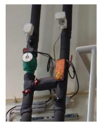
Figure 1.17. Bypass zone of the circuit.
