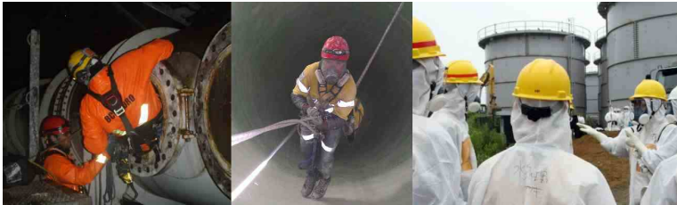
Figure 2: Inspection work by conventional methods, where it is possible to see the difficulties and dangers involved.
