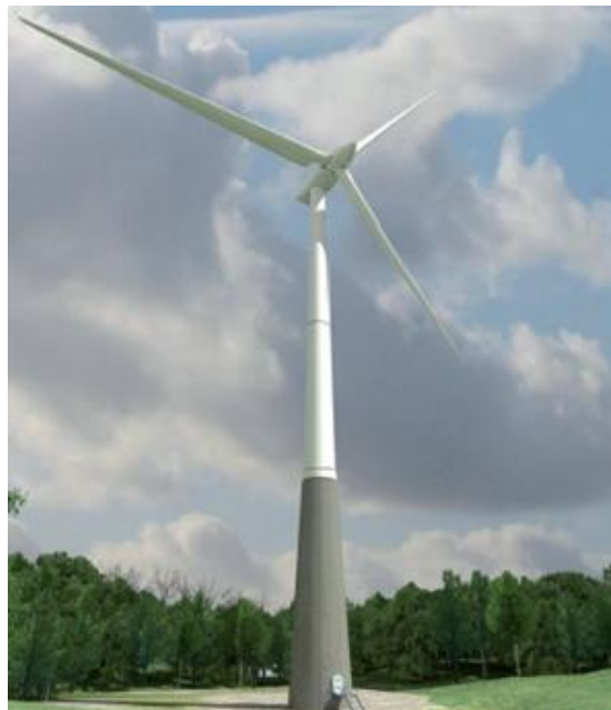
Figure 4. Concrete-steel hybrid tower.
