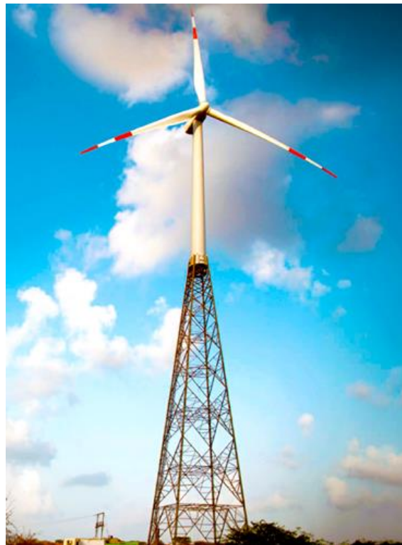
Figure 6. Hybrid lattice-tubular tower.
