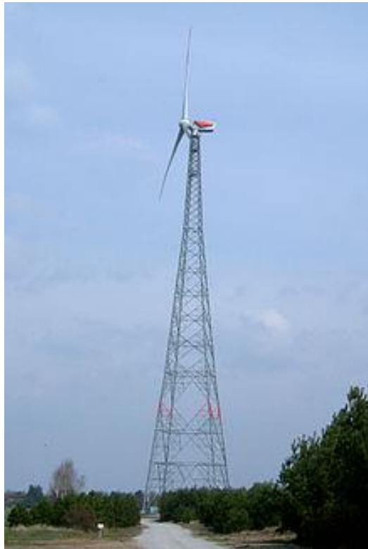
Figure 2-5 - Lattice tower of the Fuhrländer W2E (Hau, 2013)
