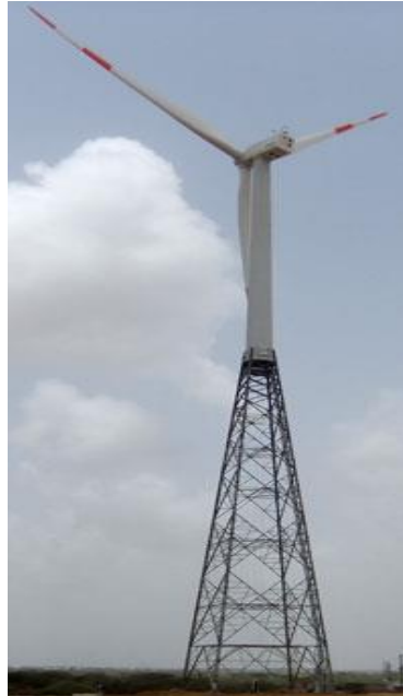
Figura 2-6 - Suzlon Hybrid Lattice-Tubular Tower ( www.suzlon.de )
