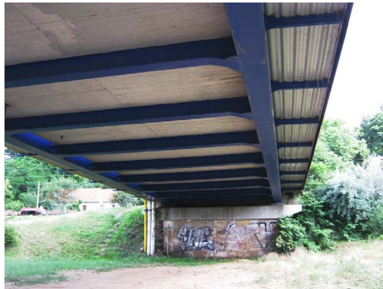
Figure 1.1 Composite bridge in Dobřichovice, Czech Republic
