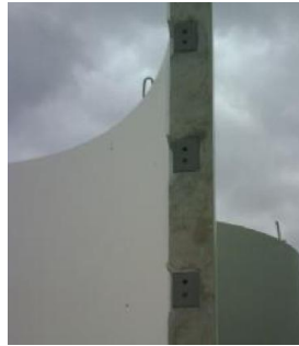
Figure 4.4 – Vertical joint in a tower segment
