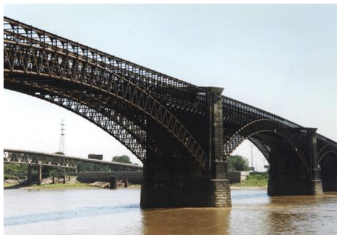
Figura 2.2 – Eads Bridge (Built St. Louis, 2013)
