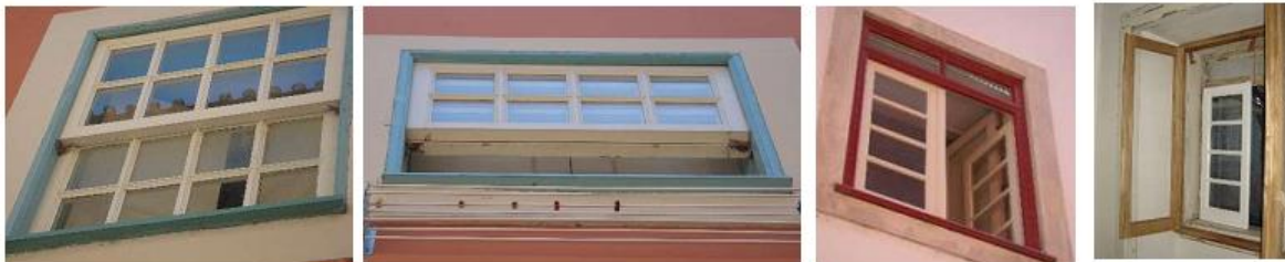
Figure 115: The properties of existing windows in Portuguese construction in Coimbra
