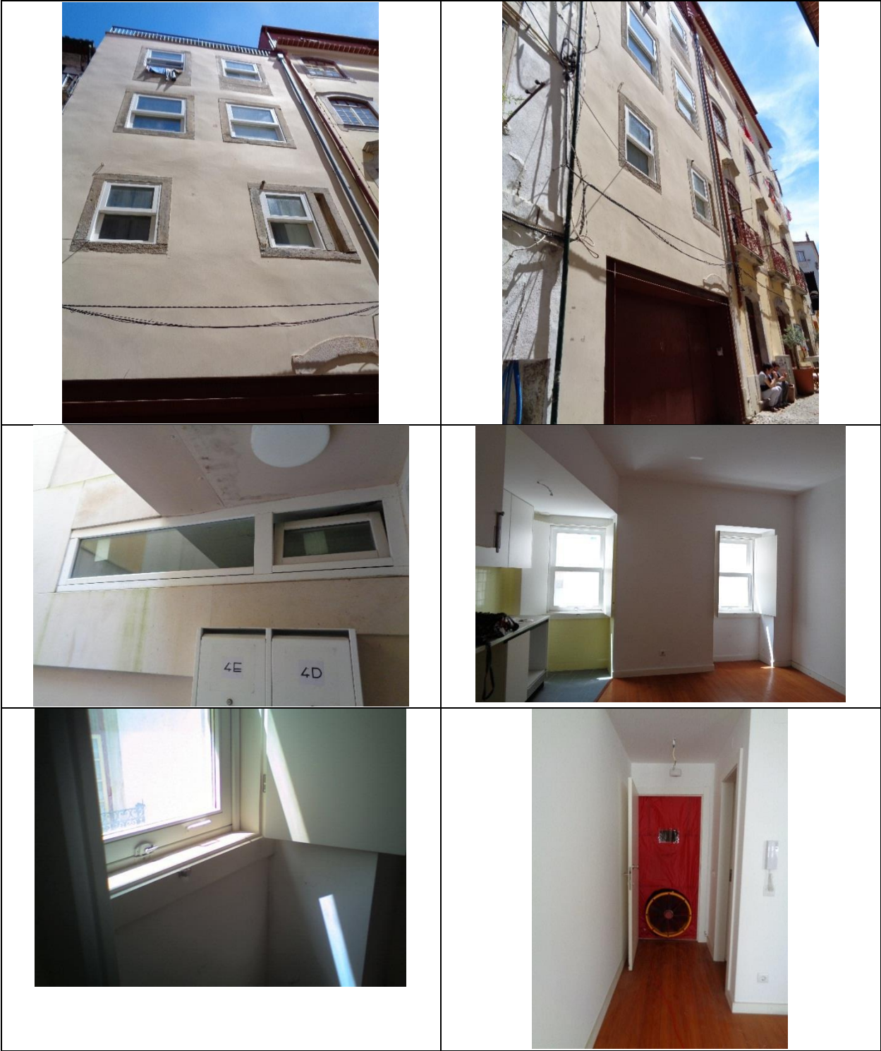
Figure 158: Interior and exterior properties of windows of the apartment. Also the procedures of BDT in the third case study
