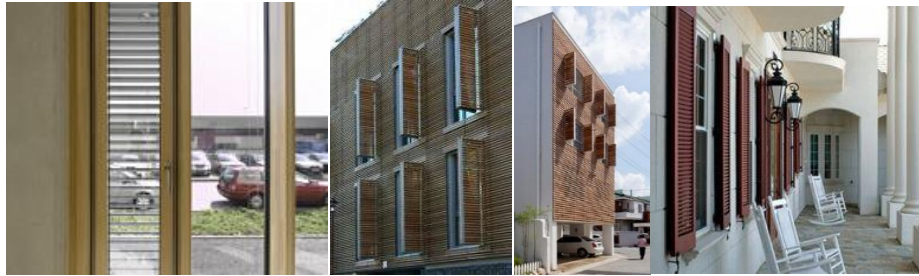
Figure 114: Window-vent surface in front of the window
