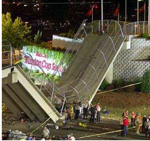
Figure 6.2: Concorde bridge collapse due to pitting corrosion (Faber, 2005).
