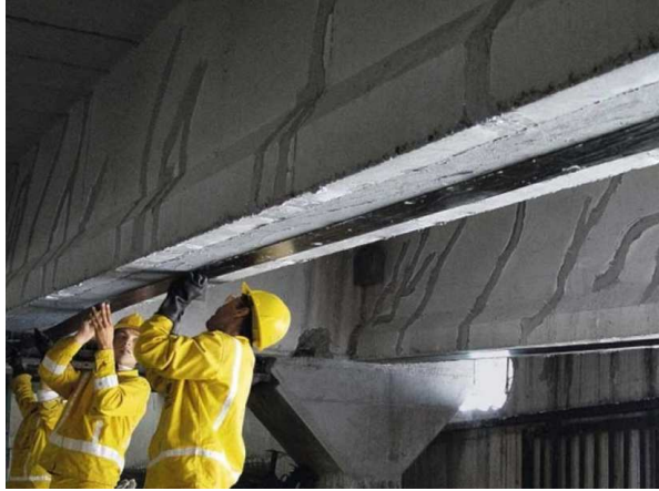
Figure 1.3: Application of FRP laminates in PC girders (Sika Group [online]).
