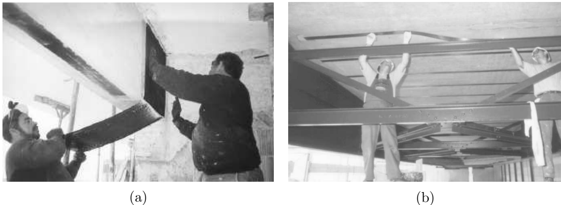
Figure 3.4: FRP application process of: (a) sheets (CEB/FIB, 2001); and (b) prefabricated laminates (Leeming and Hollaway, 1999).
