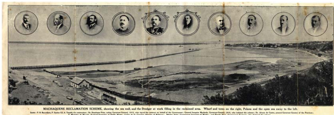
Figura 58: “Machaquene Reclamation Scheme, showing the sea wall, and the Dredger at work filling in the reclaimed area. Wharf and town on the right, Polana and the open sea away to the left. Inserts: P. B. Buccellato, P. Santos Gil, A. Tonetti, the contractors ; Dr. Domingos Frias, acting Governor-General, 1915, who signed the contract on behalf of the Government ; General Joaquim Machado, Governor-General, 1915, who initiated the scheme ; Dr. Alvaro de Castro, present Governor-General of the Province ; T. Monteiro de Macedo, Engineer-Inspector of Public Works ; Carlos de Sa Carneiro, Director of Railways ; Ribeiro Artur, Government Inspector of Works ; and Duarte Viega, Government Engineer, who designed the scheme.” [s.d.], [s.a.], CEDH-FAPF.
