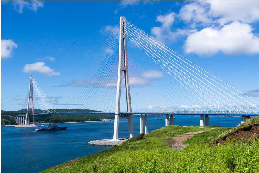
Figura 2.8 – Ponte Russky Island (Rusbridge, 2015)
