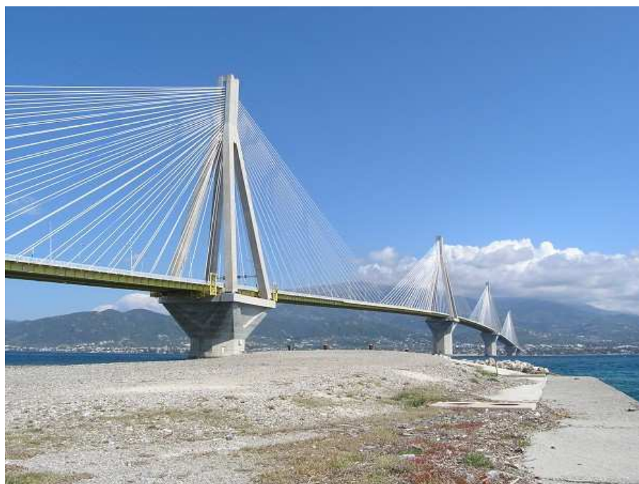
Figura 2.16 – Ponte de Rion-Antirion (Structurae, 2013)
