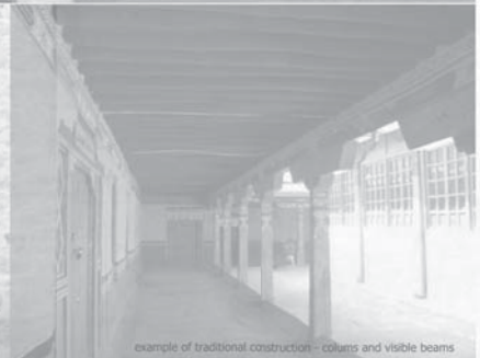
example of traditional construction - columns and visible beams
