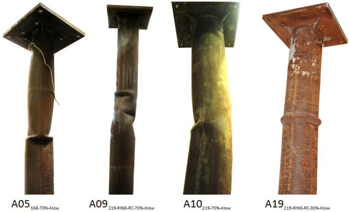
Figure 3.50 – Local buckling in tested columns.
