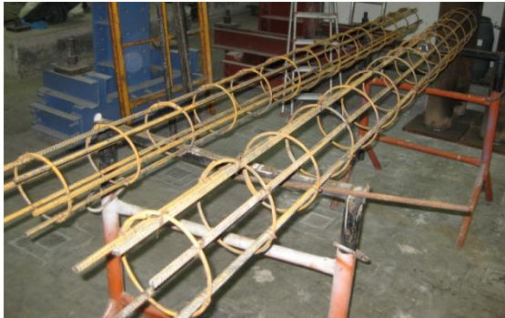
Figure 3.13 – Reinforcing steel bars and stirrups (steel reinforcement).
