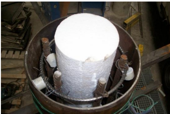
Figure 3.14 – CFCH-RC column with concrete ring before casting.
