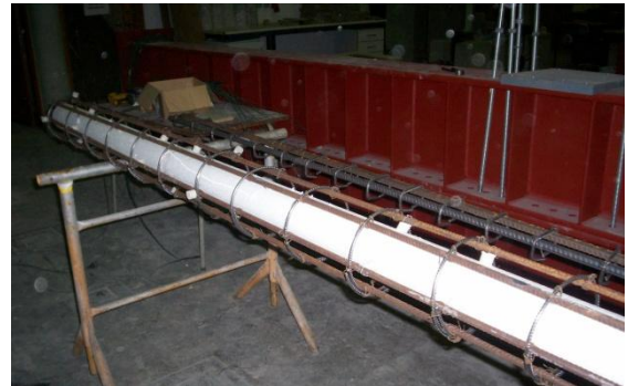
Figure 3.15 – Steel reinforcement with Styrofoam cylinder.
