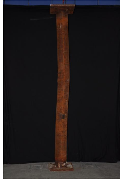
Figure D.7 – Deformed shape of column A07 219-TOT-RC-70%-Klow.
