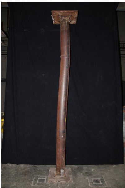
Figure D.2 – Deformed shape of column A02 168-TOT-RC-70%-Klow.
