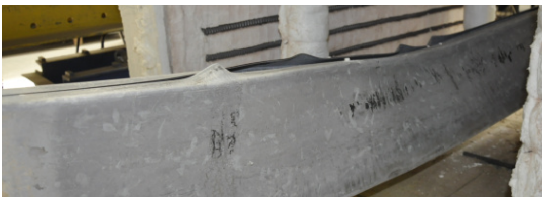
Figure F.46 – Detail view of the failure mode of the specimen B-2R_3
