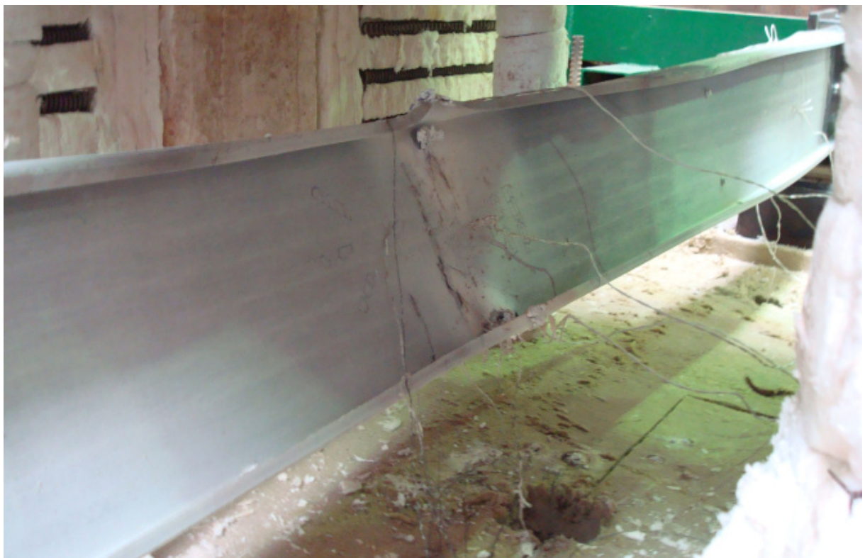
Figure F.61 – Detail view of the failure mode of the specimen B_ka-I_2
