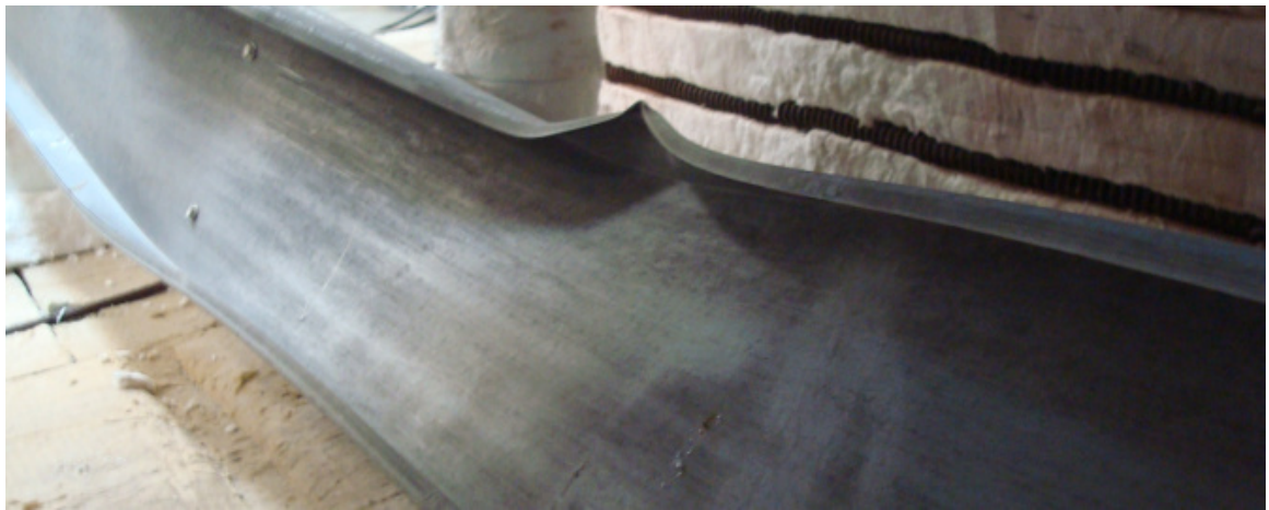
Figure F.16 – Detail view of the failure mode of the specimen B-I_1
