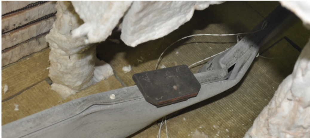
Figure F.30 – Detail view of the failure mode of the specimen B-R_2
