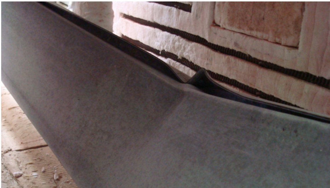
Figure F.34 – Detail view of the failure mode of the specimen B-R_3
