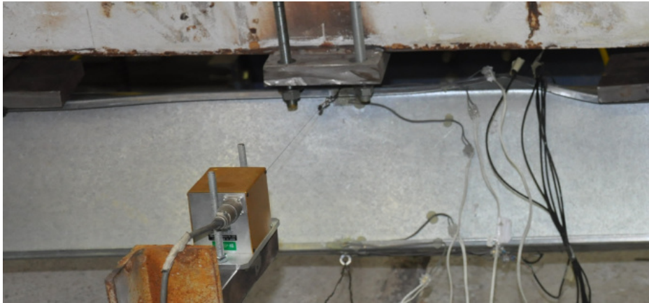
Figure B.14 – Detail view of the failure mode of specimen B-I_2
