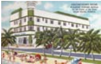
Air Conditioned Rooms Waldorf Towers Hotel On the Ocean at 9th Street Miami Beach, Florida Albert Anis, 1937 (imagem www.agilitynut.com )
