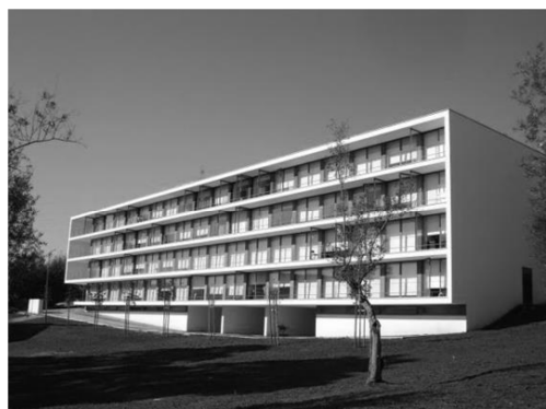
Figure 6: Student housing building, Campus II, University of Coimbra (Case study III).
