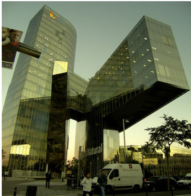
Fig 78. Torre de Gas Natural, Barcelona, Enric Miralles (1999)
